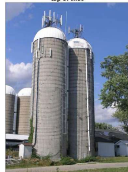
Exhibit 3-2. Two antenna arrays on top of silos
