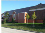
Exhibit 7-2. A loading dock screened from view by a solid wall integrated into a building's design.
