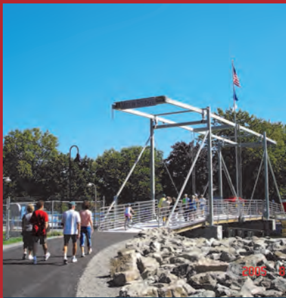
Miron Bridge Connecting the Town of Menasha & the City of Menasha
