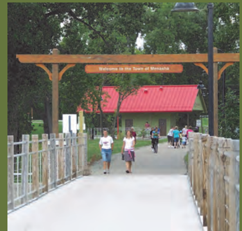
Trestle Trail Bridge
