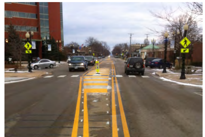
Wisconsin Ave, Neenah - Photo Courtesy of the City of Neenah
