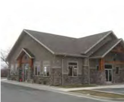
Incorporation of decorative stone and wood building materials. Pitched roofs and gables should be considered for all buildings adjacent to residential development
